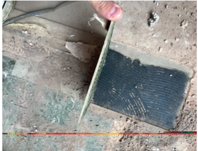
Figure 2.1. Sticky bitumen under ceramic tile
