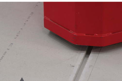
The JK Floorgrinder produces dust-free grooves in the Fermacell floor panels -
