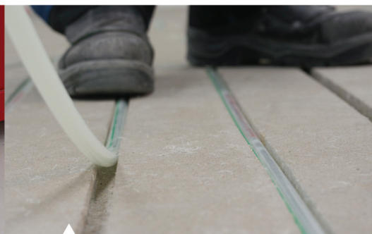
- into which the heating pipes are laid
